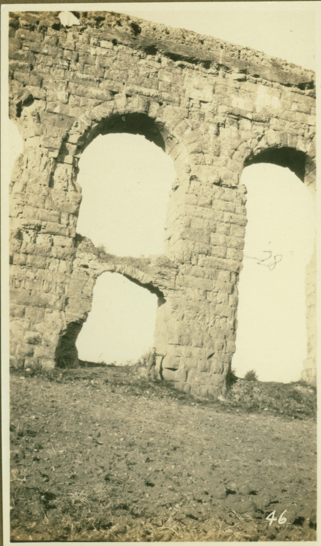
46. Ancient Aqueduct, Rome.
