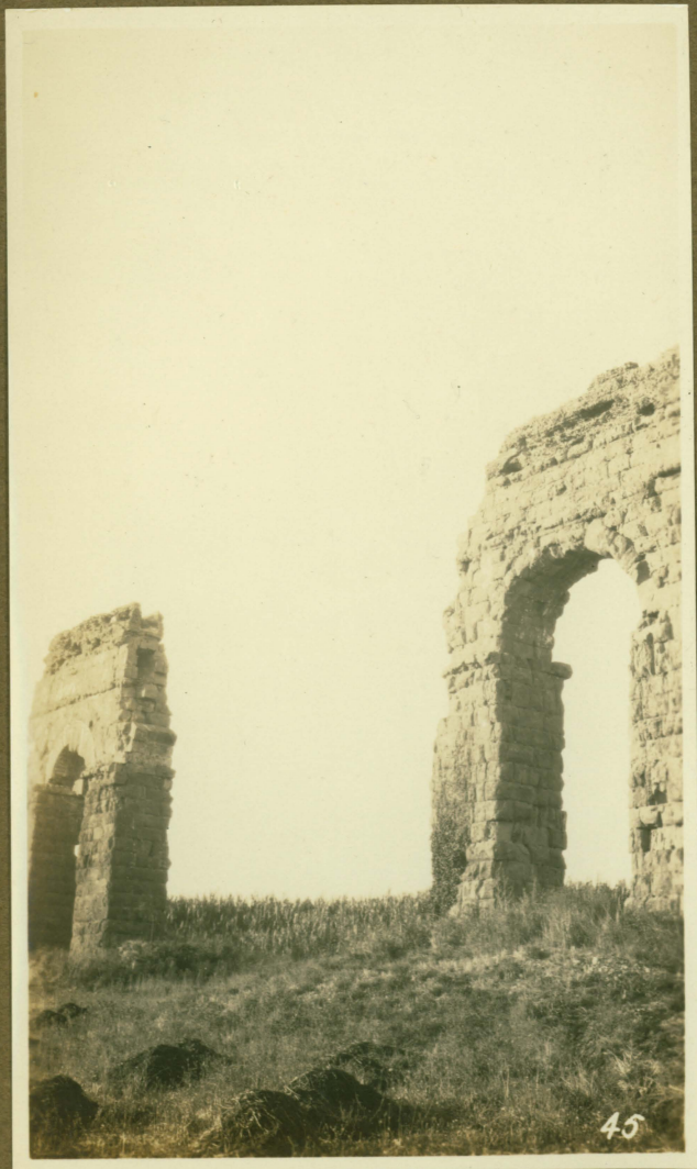
45. Ancient Aqueduct, Rome.
