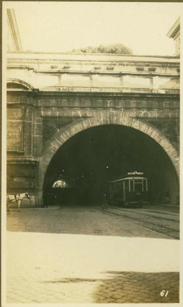
51. Tunnel in Rome.
